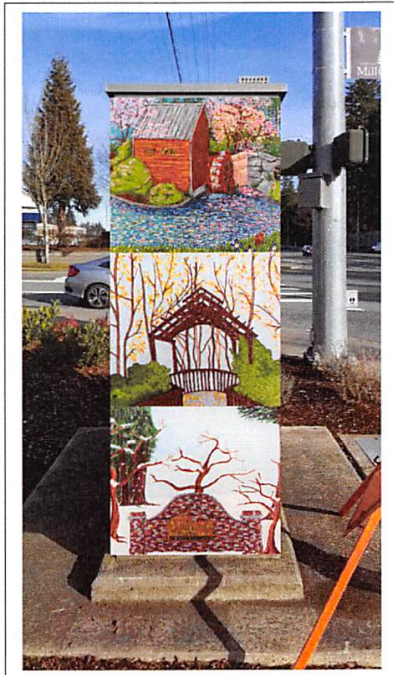
Set of three images to be used on the south-facing side of the utility boxes
